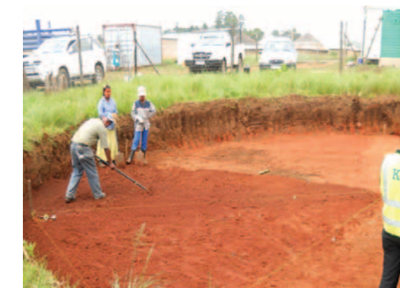
Setting out of a reservoir
