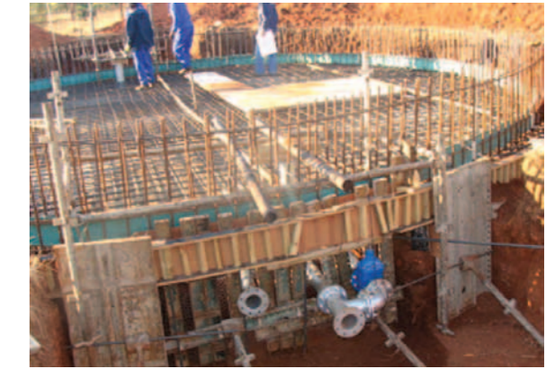
Steel fixing of a reservoir under construction
