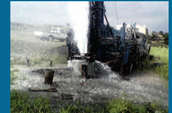
Water strike while drilling
