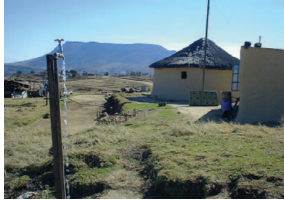
Potable water on tap
